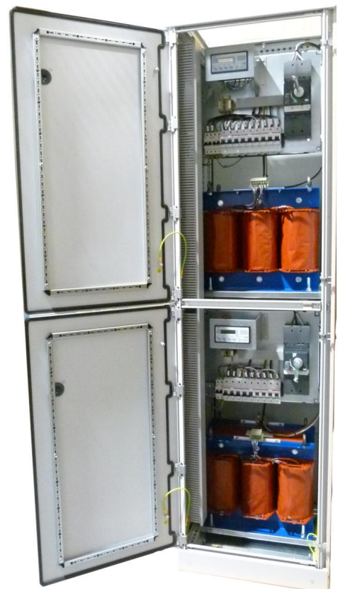
Custom-built control panel
